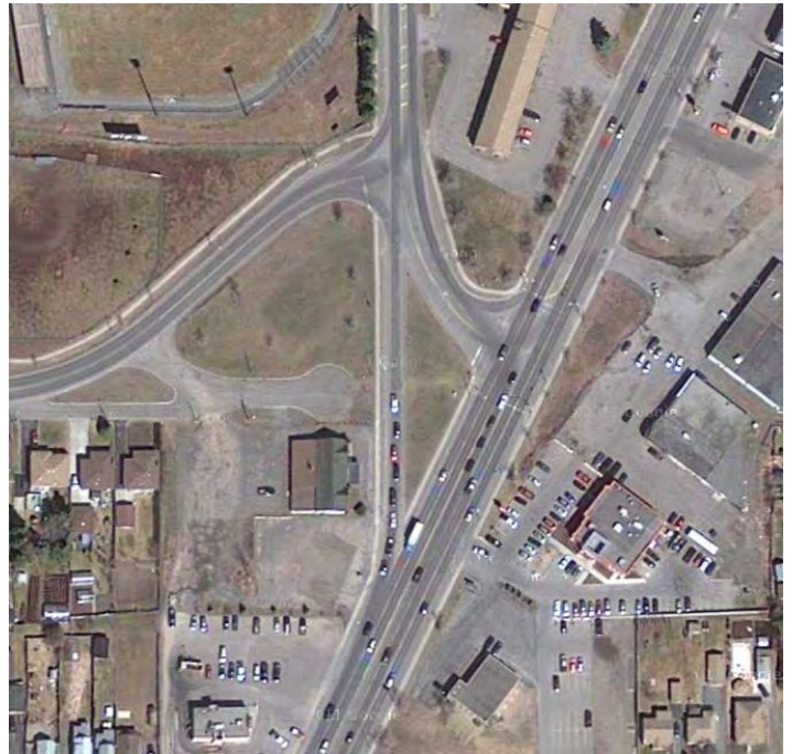
Memorial Avenue & High Street - existing condition
