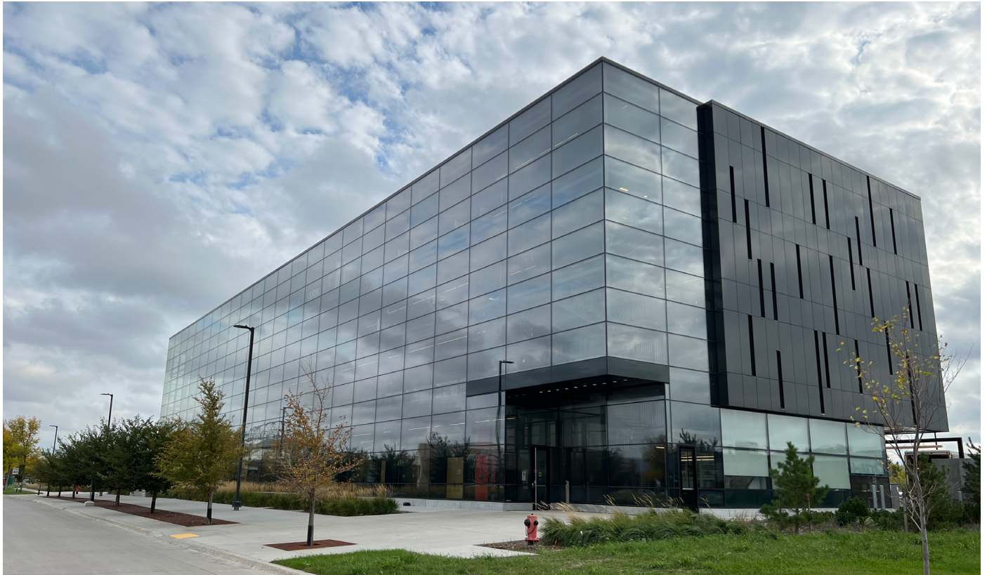
There should be no parking between the street and the primary façade.
